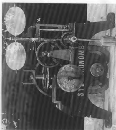
The South Brisbane Town Hall tower clock's mechanism before installation. Photo by A.G. Jackson.
