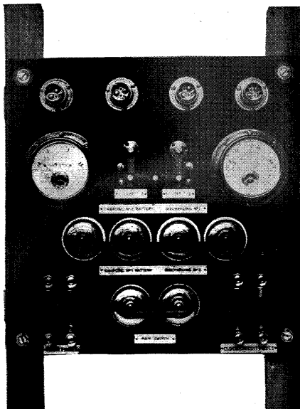
Fig. 2154.—Charging Board for Clock Circuits.
