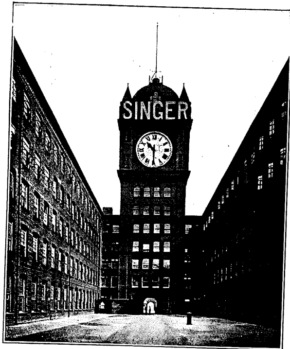
The Singer Clock Tower Operated by "Waiting-Train" Movement. For an interior view of the dials see page 20.
