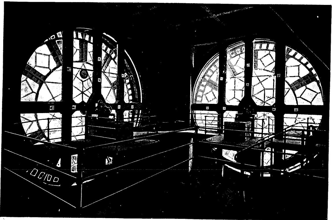
INSIDE THE CLOCK CHAMBER, ROYAL LIVER BUILDING, LIVERPOOL. Shewing the Two Bases for Two of the Waiting Train Movements.
